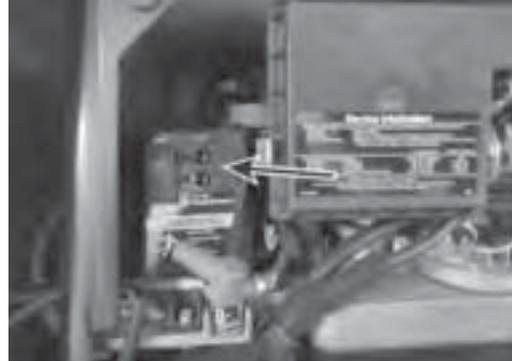
*The output from the generator may be interrupted if the main generator circuit breakers trip. These breakers are located on the main generator control panel. If there is no power when the generator is running, check and reset these breakers.*
