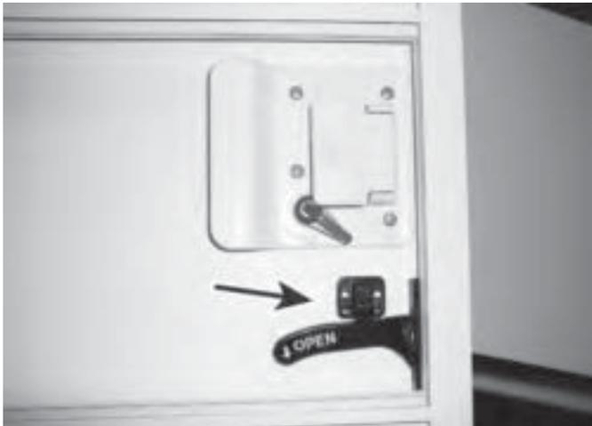
Adjust the screen door latch by loosening the screws as shown. Move the latch plate for a good fit when the screen door is closed. Tighten screws after adjustment.
