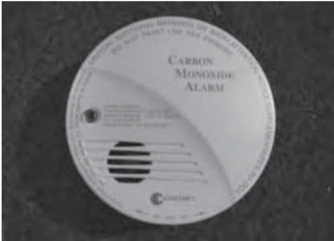
A battery-powered carbon monoxide (CO) detector/alarm is installed in or near the main sleeping area. Detailed operating and maintenance instructions are in the Owner's Information Packet.
