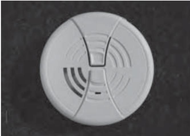
A battery-powered smoke detector is mounted on the ceiling in the living/cooking area of the trailer. Detailed operating and maintenance instructions for the smoke detector are in your Owner's Information Packet.
