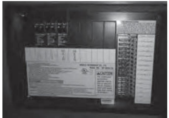
Under low voltage, fuses and circuit breakers can blow without a short circuit condition. The refrigerator control system requires at least 10.5 volts and will shut down even with propane supplied, potentially ruining food in the refrigerator.
