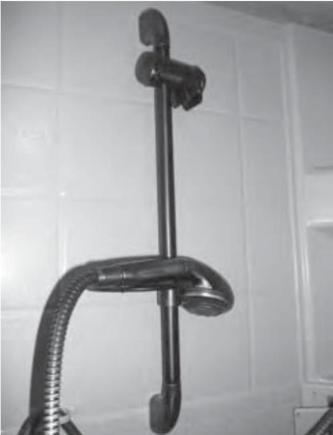
Open all faucets, both hot and cold, in the galley, bathroom and shower. Open the shower head valve. This will allow the water in the lines to flow to the low point drains.
