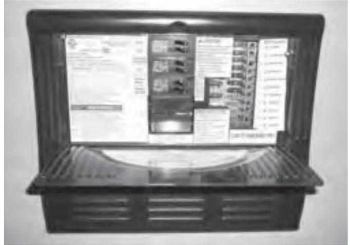
Your trailer is supplied with a converter. The converter converts 120-volt AC current to 12-volt DC. It provides DC power to operate the DC electrical system and charge the batteries.
