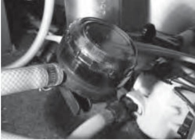
Cleaning the fresh water pump inlet filters is a normal customer maintenance item. It is normal for debris to collect in this filter, especially during the first use of the plumbing system. It is performing its function by trapping any minor debris which might be present in the water. The water pump is typically mounted to the floor inside the unit inside the kitchen base. Removing drawers usually exposes the pump.
