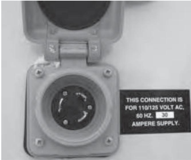
When connecting the cord to the service, push the plug straight into the receptacle until it seats completely.
