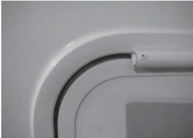
While washing, make note of any maintenance that may be needed. Closely inspect the sealants around roof accessories (vents, antennas, racks, etc.), windows and doors. Reseal as necessary before winter rains or snows accumulate.
