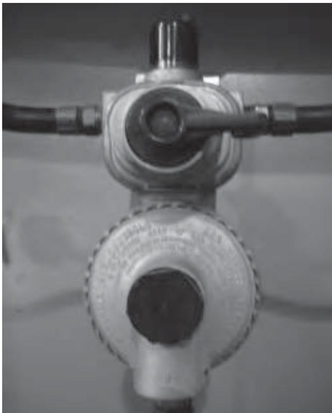
2. Loosen the hand nut attaching the flexible hose to the cylinder.
